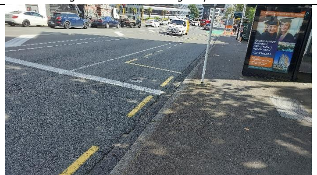
Pavement and carriageway detail S of
