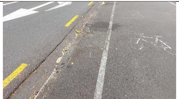
Detail showing Pavement and carriageway
