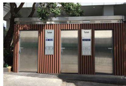
Exeloo Orbit - Lower Albert Street Auckland Consideration of level tie in to accessible unit from sloped footpath.
