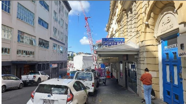
Looking S towards Mercury Lane Theatre entrance
