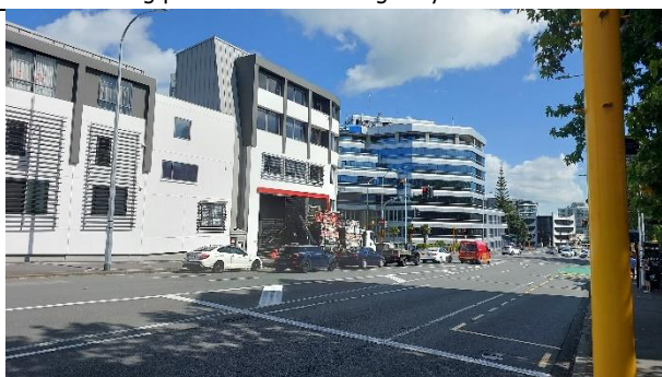
Looking NW towards Hopetoun St Junction
