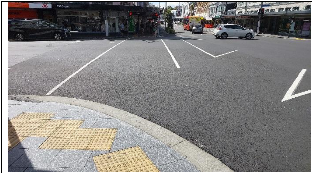
Recent paving treatment at Junction Karangahape Road
