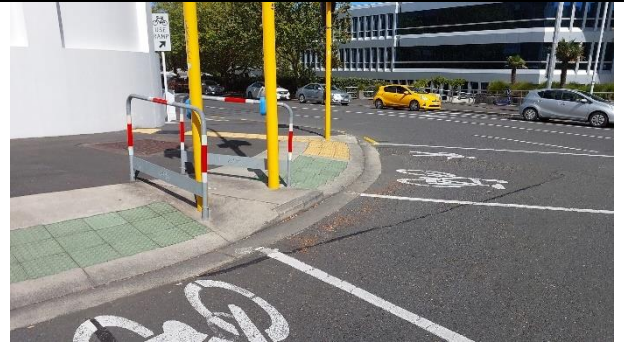
Existing ground treatment at Junction with Hopetoun Street Looking NW
