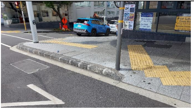
Recent paving and road surfacing at Mercury Lane with reused kerbstones
