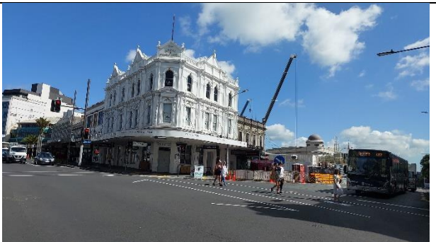
Looking NW from Mercury Lane
