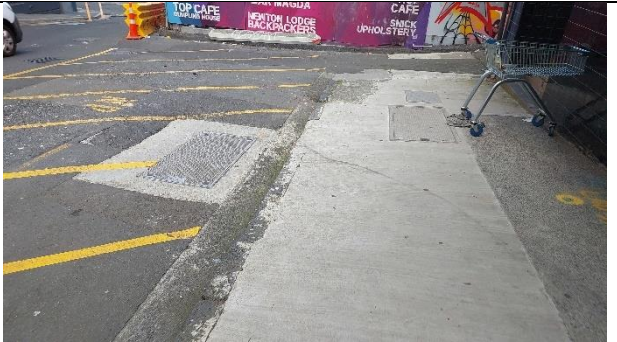
Typical Paving treatment
